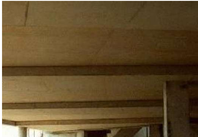
One way slab with band beam
