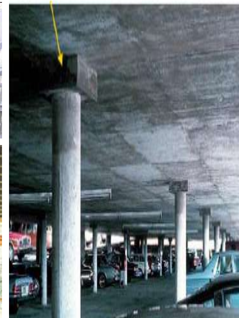
Flat slab w drop panel
